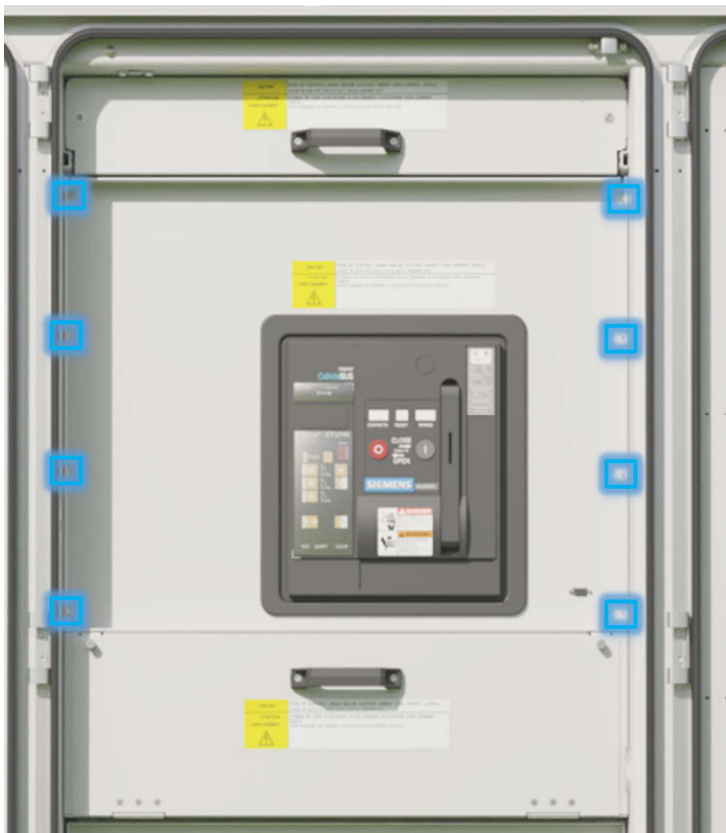
Figure 93. Removing Circuit Breaker Panel
