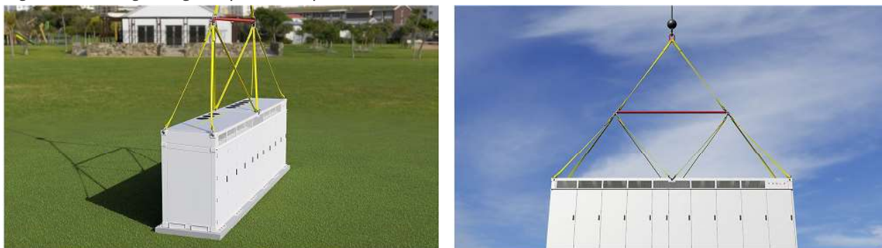
Figure 75. Lifting Using Straps and a Spreader Bar
